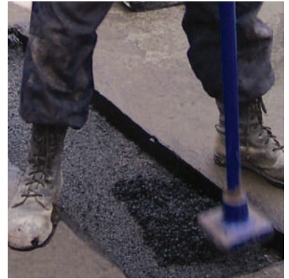
Tamp down with Tarmac Tamper for a smooth professional finish
