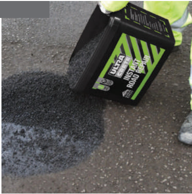
Remove debris from hole and fill with Instant Pothole Repair
